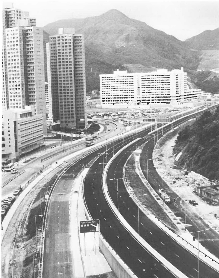
New Territories Circular Road — Shatin section that will link Lion Rock Tunnel Road and Tai Po Road at the Shatin race course when completed in mid-1985.
