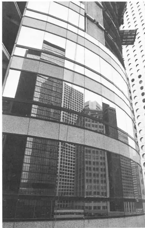
Hong Kong's central business district is dramatically reflected in Exchange Square's new cladding as alternating bands of rose-coloured granite and silver glass appear on the development's exterior.
